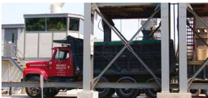
Integration of truck scale operations with filling or load-out systems
